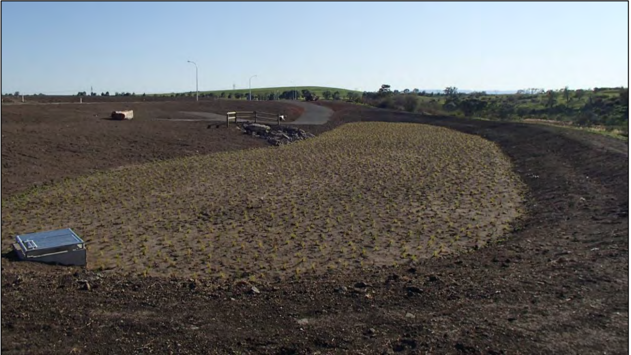
Figure 7: North Park Estate Bio-Retention System following construction of the treatment asset
