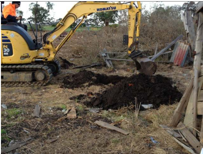
PLATE 4 Test-pitting within the cleared asbestos area.
