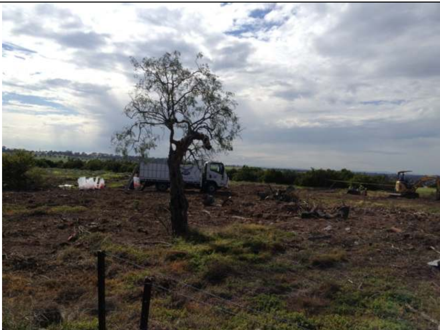
PLATE 2 Looking north-east over the "exclusion zone" area of asbestos clearance.
