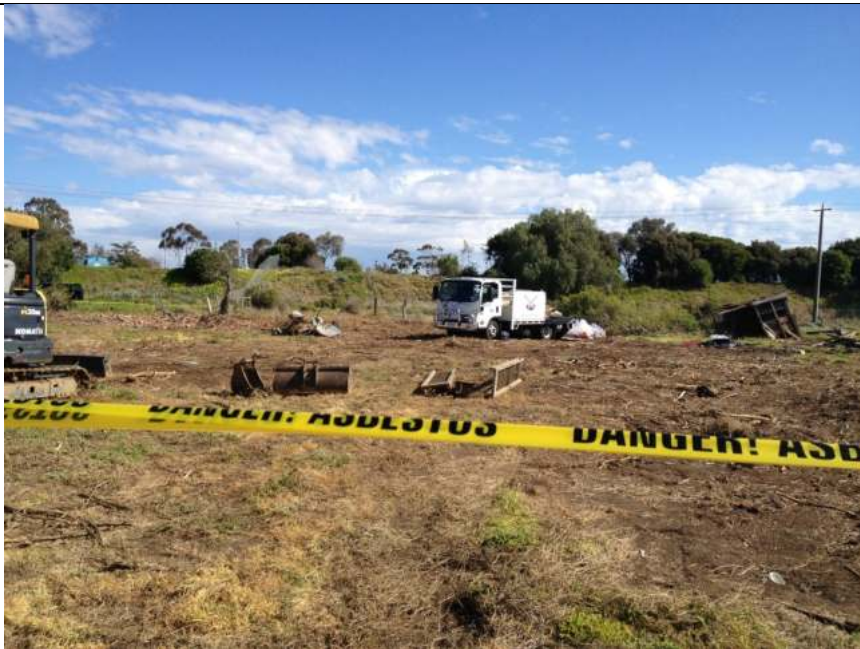
PLATE 4 Looking north-west. Asbestos clearance works progressing.
