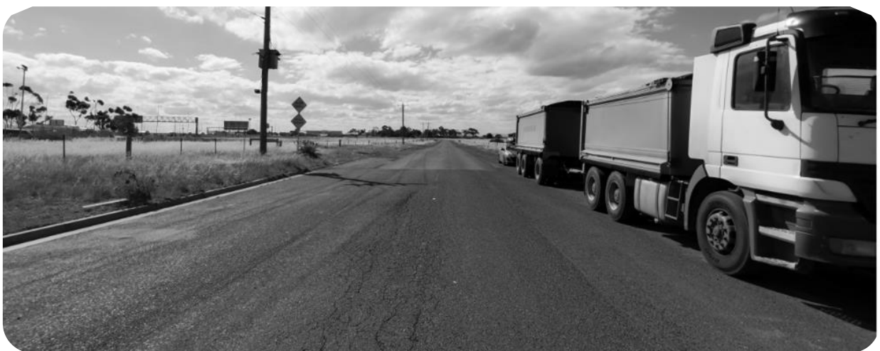
Figure 3 Western Avenue carriageway, facing west of Wright Street
