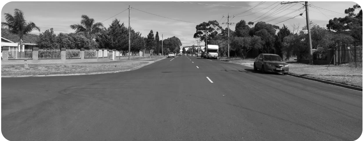
Figure 2 Western Avenue carriageway, facing east past Wright Street
