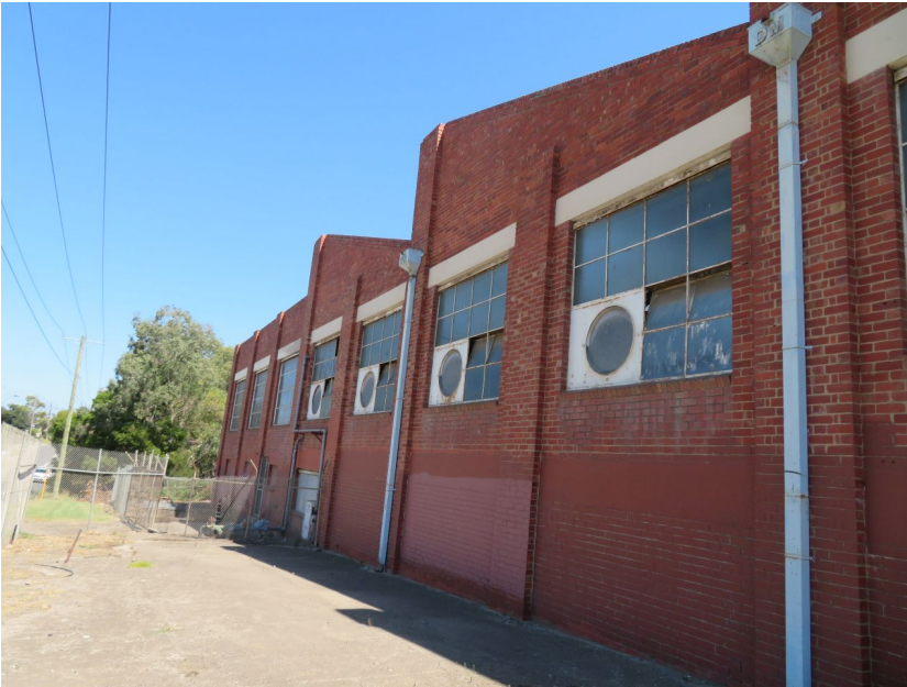
Figure 14 View from the southern end of the east elevation, showing multi-paned windows with alterations
