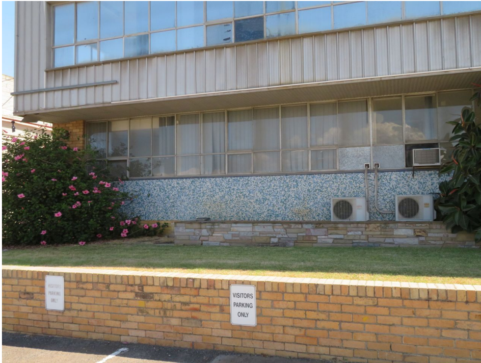
Figure 19 Detail of the mosaic tiling plinth, Castlemaine stone planters and brick retaining wall
