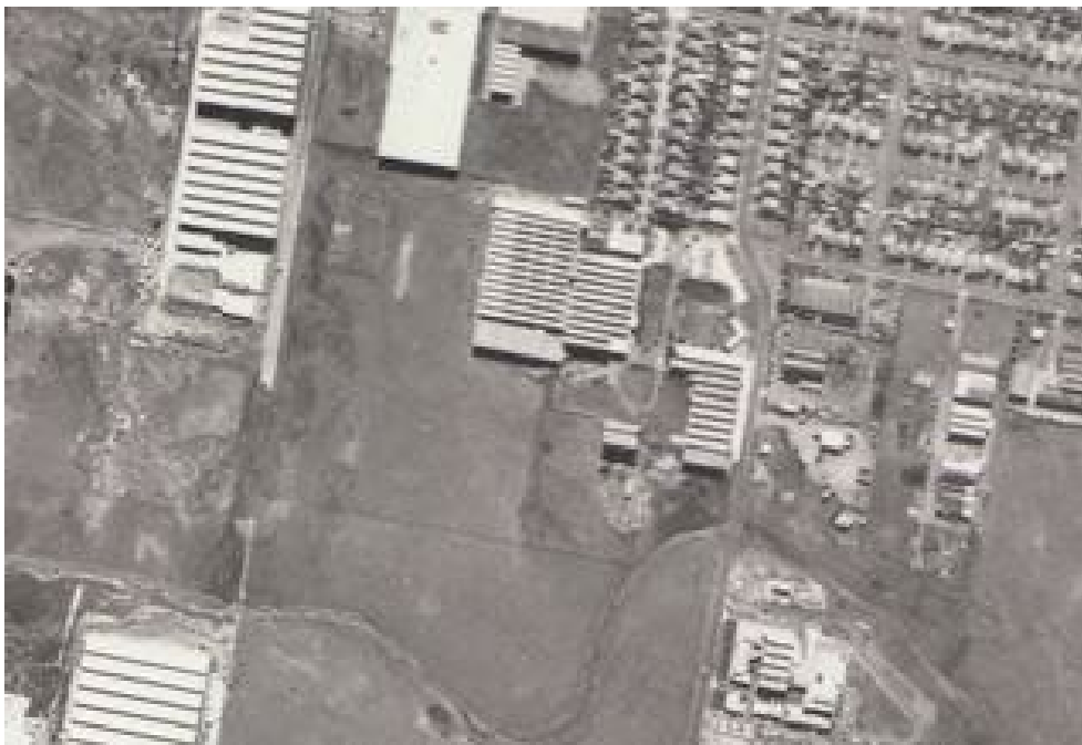
Figure 6 1966 aerial photograph of the subject site Source: Landvic
