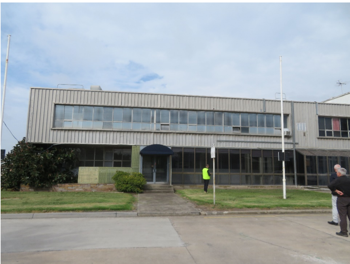
Figure 18 North elevation of the administration block (Building G)
