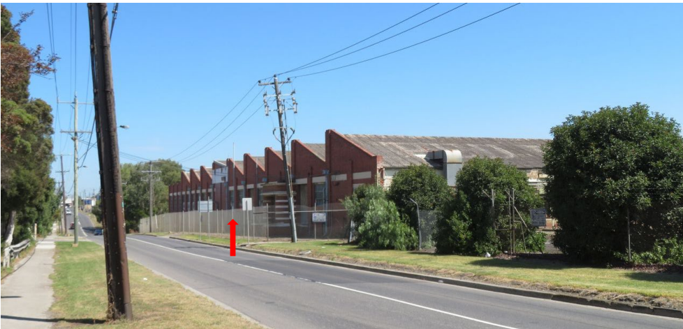
Figure 15 View of the Building E sawtooth form from Paramount Road, entrance portico indicated
