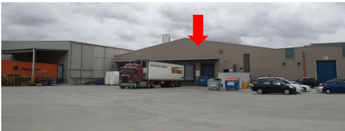
Figure 10 South side of Building B (indicated), south side of Building C to right of image
