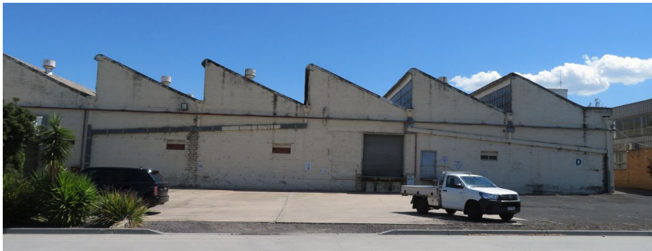
Figure 13 Building D east elevation
