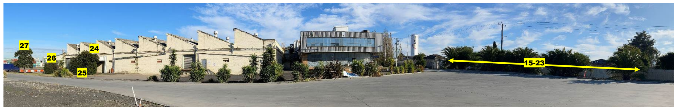
Image 3: Looking west at warehouses of Paramount site. Trees 15 – 27.
