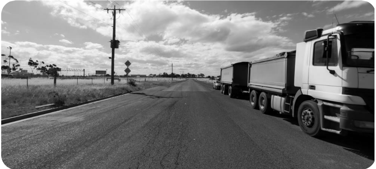
Figure 3 Western Avenue carriageway, facing west of Wright Street
