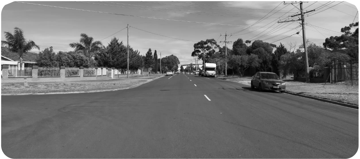
Figure 2 Western Avenue carriageway, facing east past Wright Street
