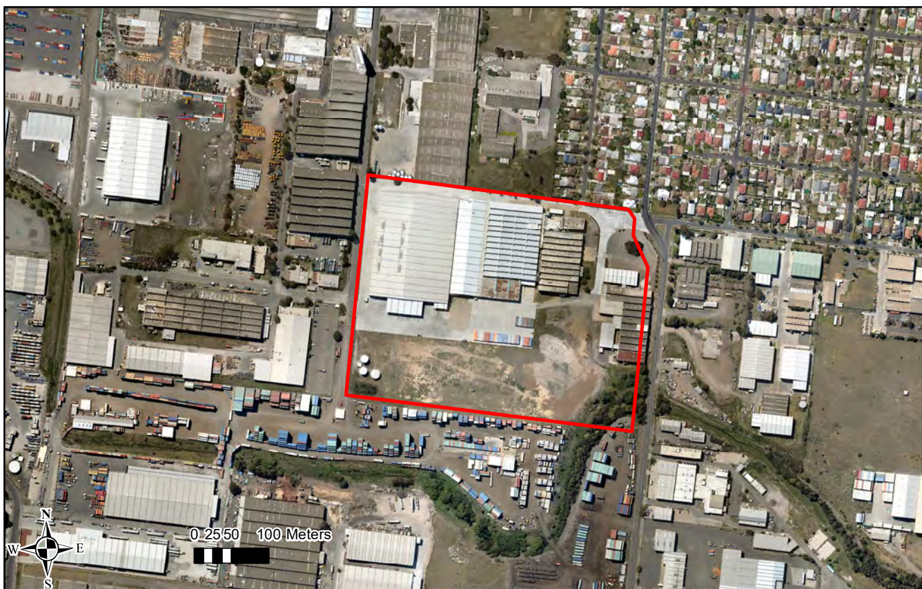
Aerial Photograph of Site (2009) Job Number: J164174
