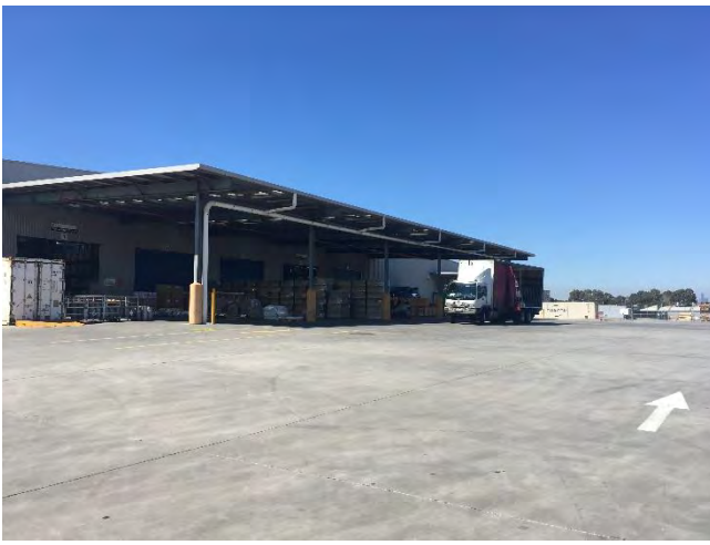
Overview of the site, facing north east
